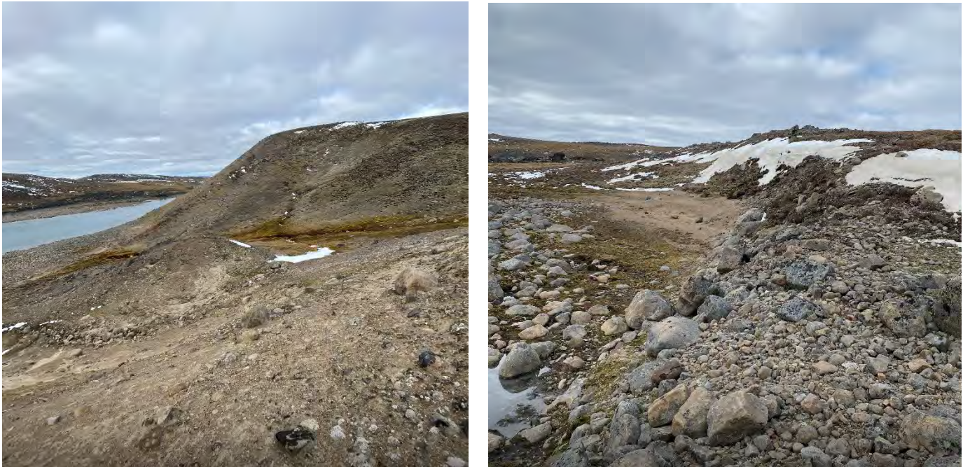
Images 6-11 and 6-12: Northwest views of the East Alignment on Line X3
